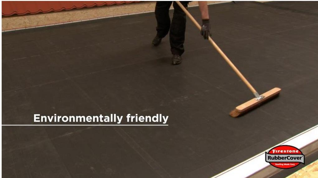
It is important to make sure you firmly adhere the EPDM membrane properly to the roof deck once the adhesive has become tacky. Use a wide-span domestic broom with soft bristles to press down the membrane, the roller to push out any bubbles, and the penny roller into the corners and edges.
