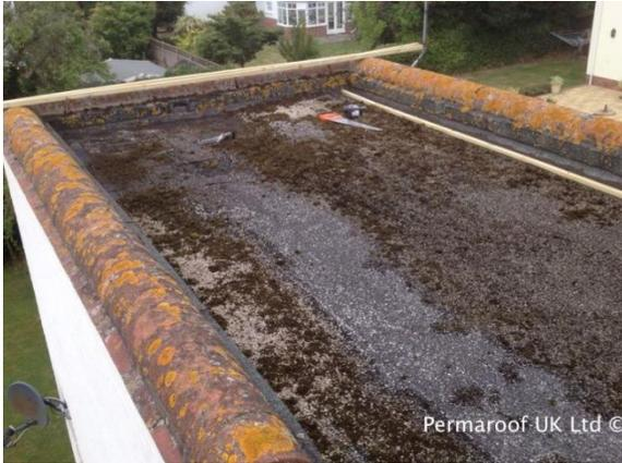
The first thing that you need to do before installing an EPDM membrane is to make sure that the roof surface is completely clean and clear.
