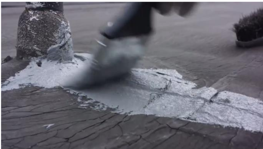
Figs 5 & 6 - Working the Emergency Roof Repair into the damaged area of the flat roof.
