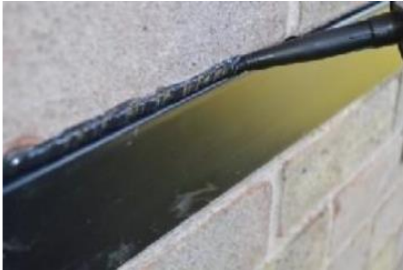
Fig 7: Sealing up the chase with Permaroof Ultrabond.
