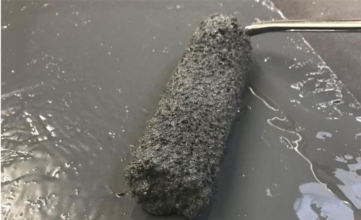
Although used widely in commercial waterproofing and professional surfacing sectors, Liquid PU (also known as rubber roofing) is also suitable for the experienced DIY market with its rapid curing time, ease of application and because it can be applied over existing flat roof coverings.
