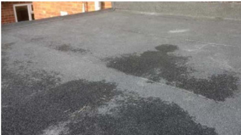
If the felt has been previously overlaid with a liquid coating and has suffered water ingress leading to delamination, remove where possible and again inspect the felt.
