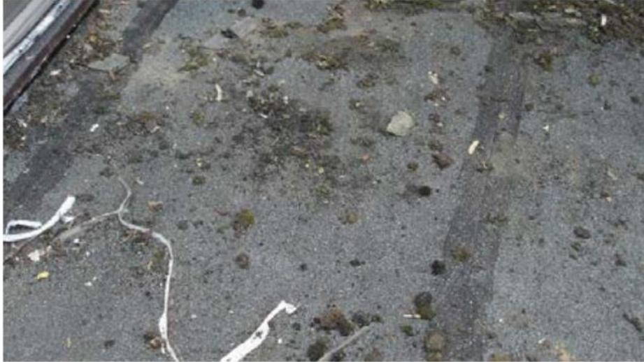
Inspect existing felt, brush any loose chippings and remove. Any bubbles or blisters, small cracks and damaged areas can be repaired with matting embedded in a coat of liquid membrane. Existing flat areas must be clean, dry and free from any contaminants such as oil, grease and dust. Thoroughly clean by power washing and allow to dry. Treat all moss/vegetation with wash treatment.
