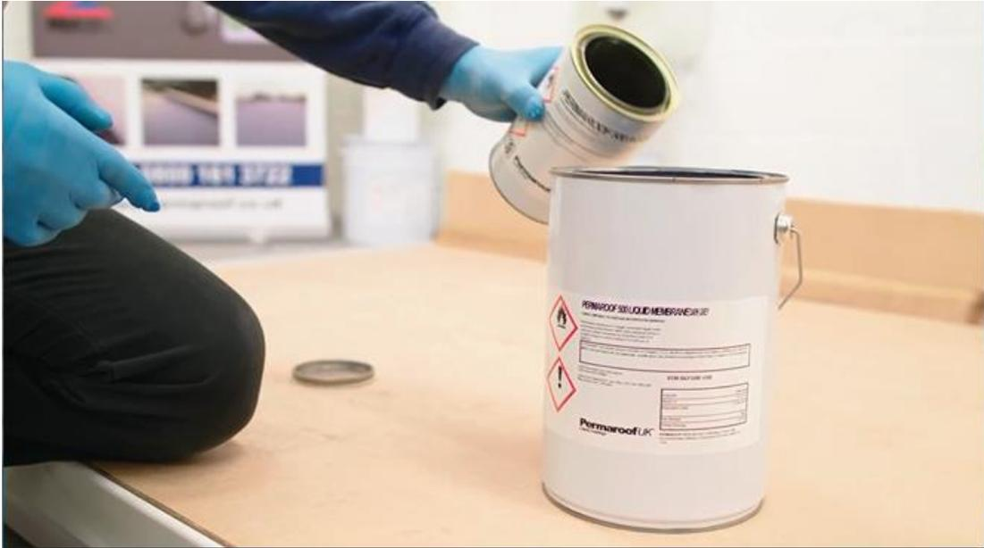
When first opening liquid membrane tins, the product must be stirred thoroughly ensuring any settlement at the bottom is mixed in. Accelerator is then added at the exact ratio of 110ml (of accelerator) per litre of liquid membrane (or 2Ltr/25kg tin or 500ml/6kg tin of liquid membrane) and mixed at a slow speed to avoid air entrapment/bubbles.
