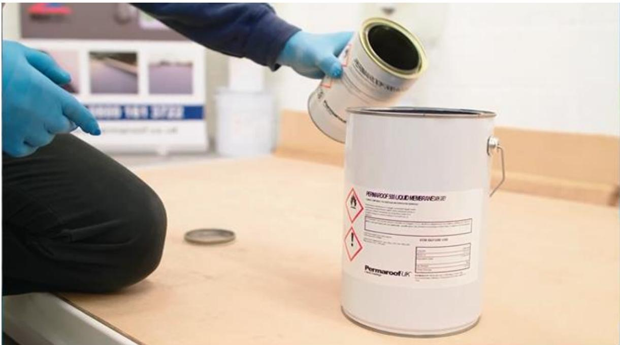
When first opening liquid membrane tins, the product must be stirred thoroughly ensuring any settlement at the bottom is mixed in.
