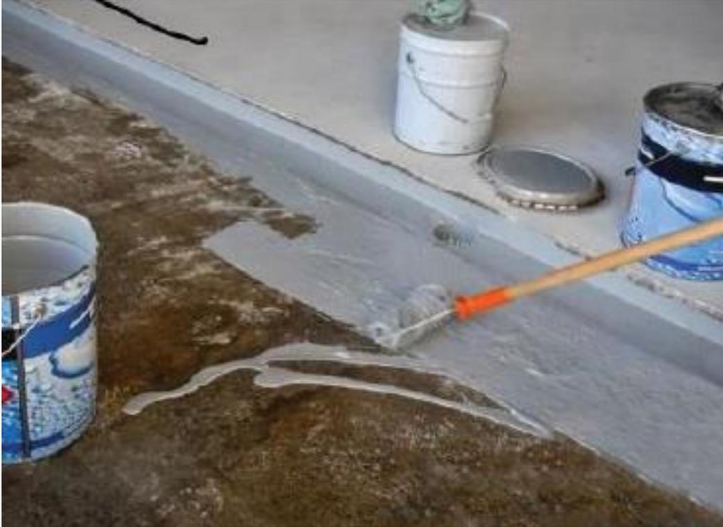
Apply accelerated liquid membrane to the whole area of the roof in one layer using a solvent resistant roller. Liquid membrane is self-levelling, do not overwork the product, it's easier to work out the coverage for the mixed tin, pour and spread by roller.
