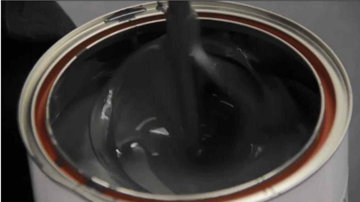
Make sure the accelerator and liquid membrane are thoroughly mixed together before applying (This should take a couple of minutes).
