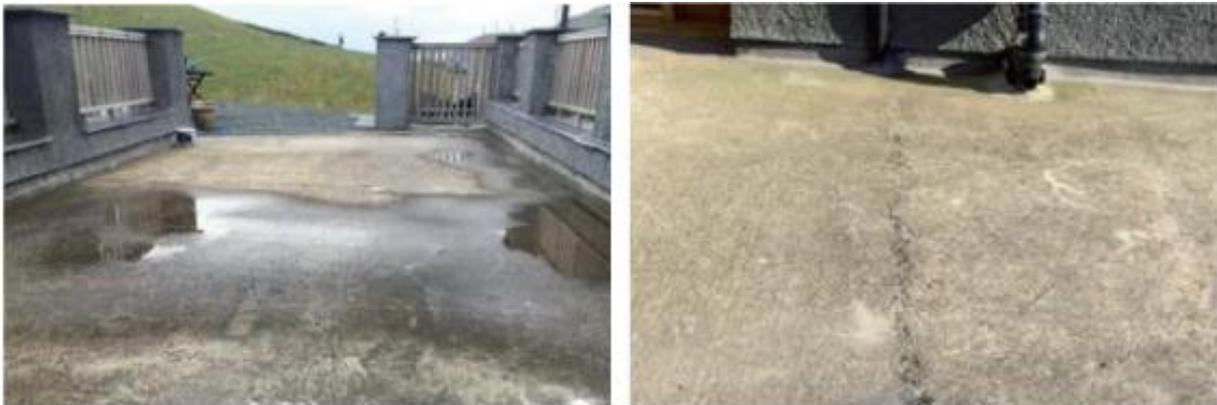
Any small cracks and damaged areas can be repaired with matting embedded in a coat of liquid membrane (AFTER PRIMING).
