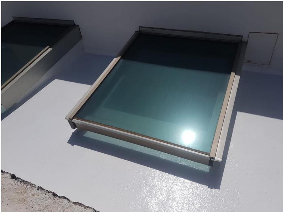
If the rooflights have been coated with another roof system, the change of material also needs to be reinforced with the matting (as above), where it meets the liquid membrane.
